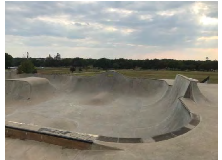
The Lockhart Skatepark is a poured-in-place concrete facility that offers a variety of vertical and street elements for skaters of all ages.
