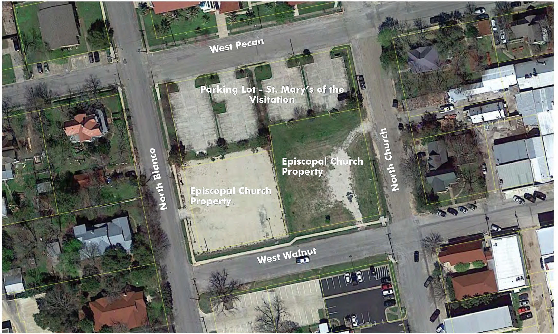
Site Aerial Photo - LOT 29 AT N. WALNUT AND N. CHURCH STREET Not to Scale
