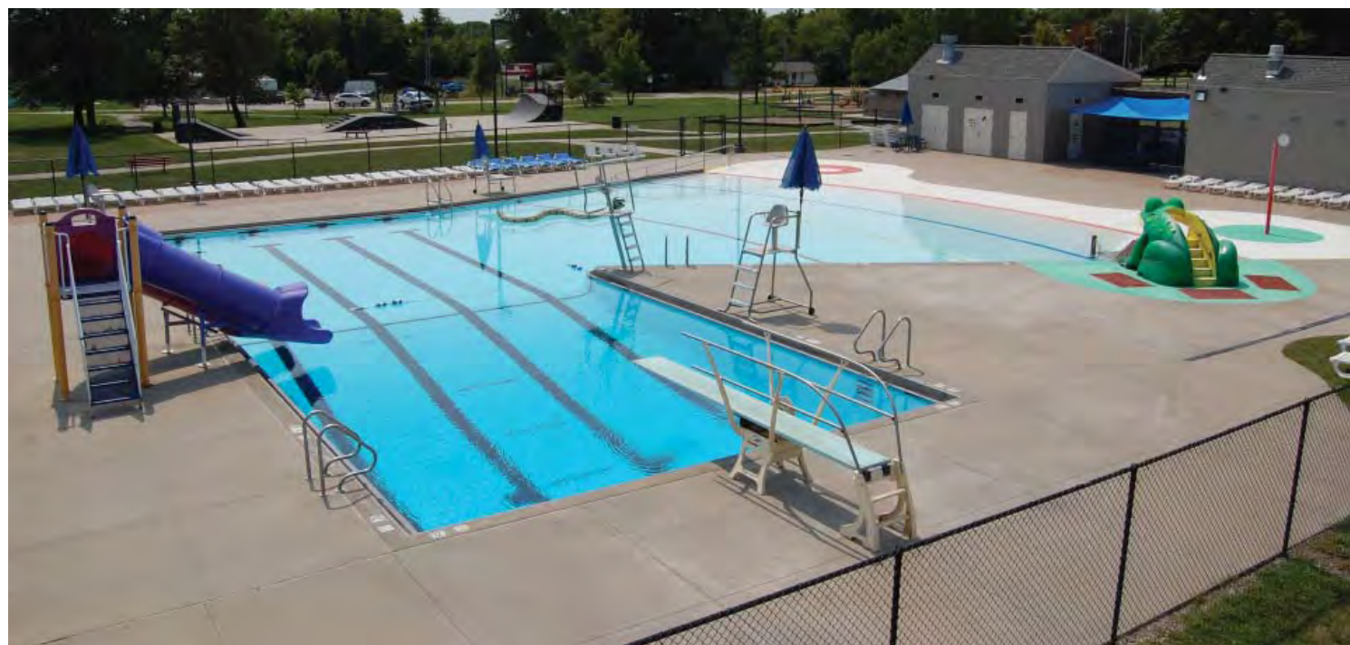
Modern zero-depth entry pools cater to a wide range of users, providing ease of access to the water for young children and senior citizens or users who may be more comfortable in shallow-water environments. Existing pools can be renovated to include this style of shallow area while retaining traditional competition/lap lanes. (source: City of Grain Valley, MO)
