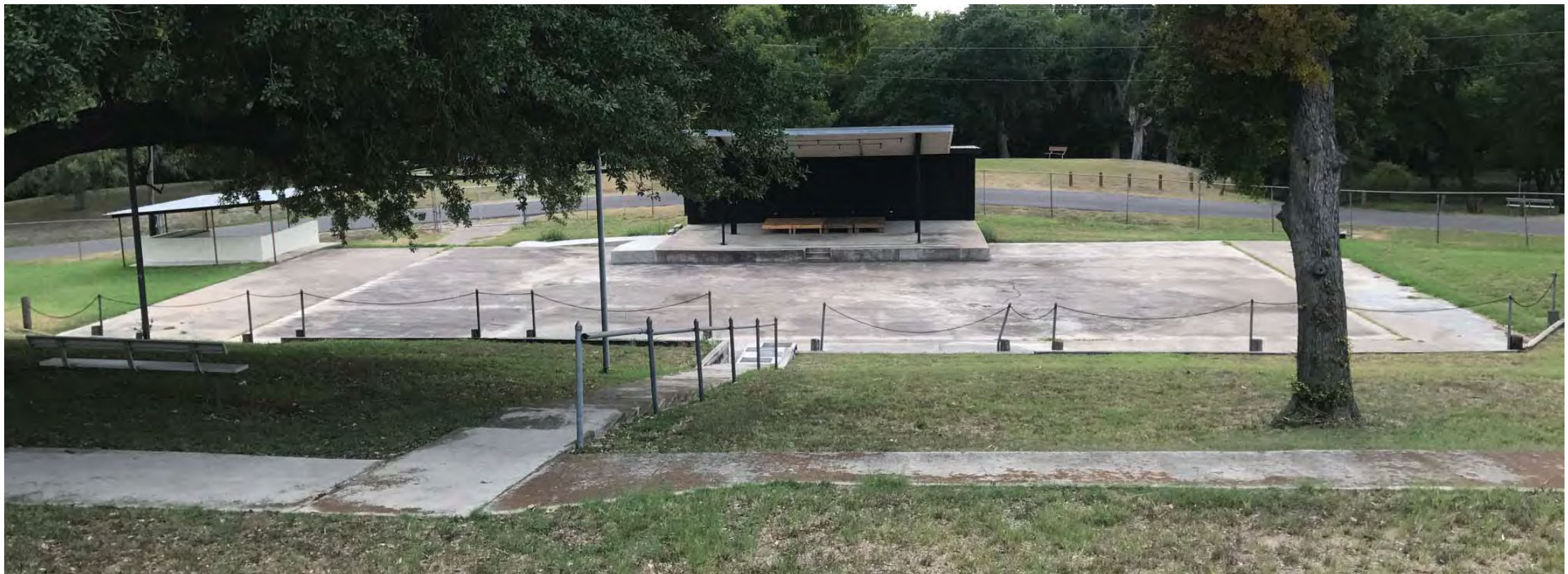
The City Park Amphitheater is home to a variety of performances and activities. Renovation of the site could create a more inviting and functional venue for promoting local music acts and recreation and economic development activities.
