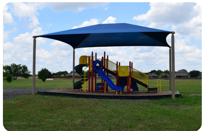
Playscape in Maple Street Park. Overall condition is average.
