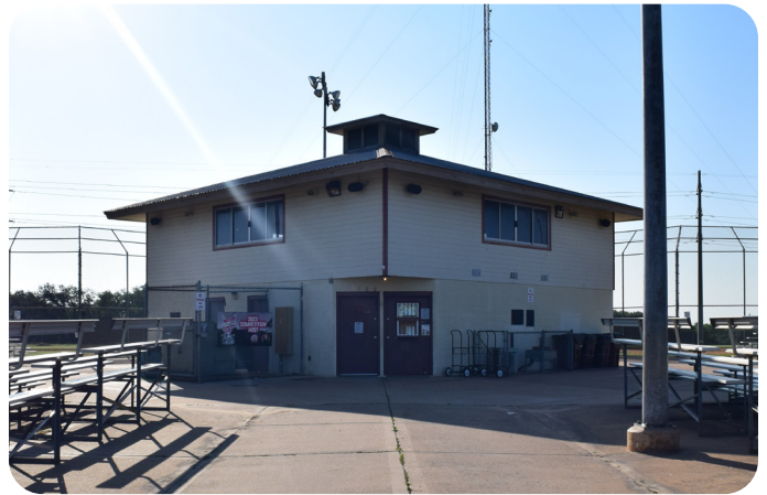
Club house at the Youth Sports Complex. Overall condition is average.
