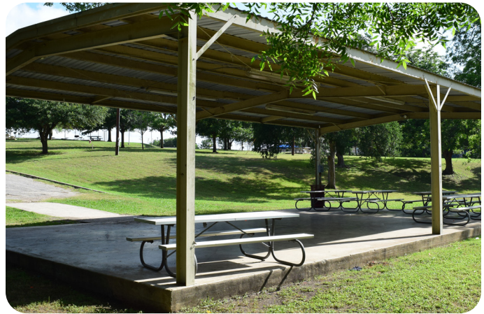
Public gathering pavilion in City Park. Overall condition is average. More seating is needed.
