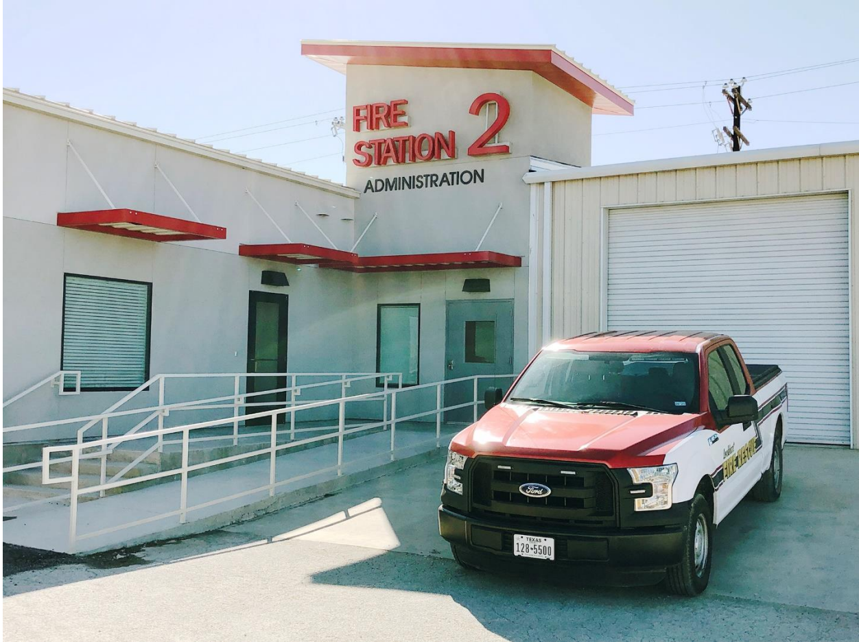
Fire Station No. 2 is located at 1911 Borchert Drive. The fire station has access points to both State Highway 142 (San Antonio Street) and Borchert Drive.
