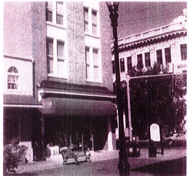
Figure 20. A dome awning was an inappropriate addition to this circa 1890s building. In order to qualify for historic tax credits the new vinyl awning was replaced with a shed awning with a canvas-like woven acrylic covering.
