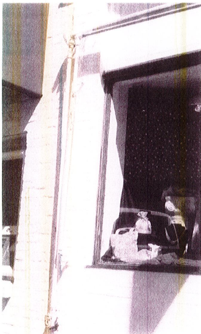
Figure 17. A gearbox, slide rod, roller, front bar, and extension arm reveal that this 19th century building once featured a retractable awning. It is likely that with minor repairs the surviving hardware could again be made operable, recovered with a canvas or acrylic fabric, and reused to service the storefront.
