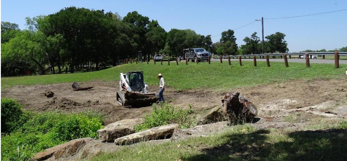
*Fig 3. Rain Garden site with City contractor preparing the “bowl” and placing large wood and rock to divert approx.. 30% of flow from the drain into the garden area.*
