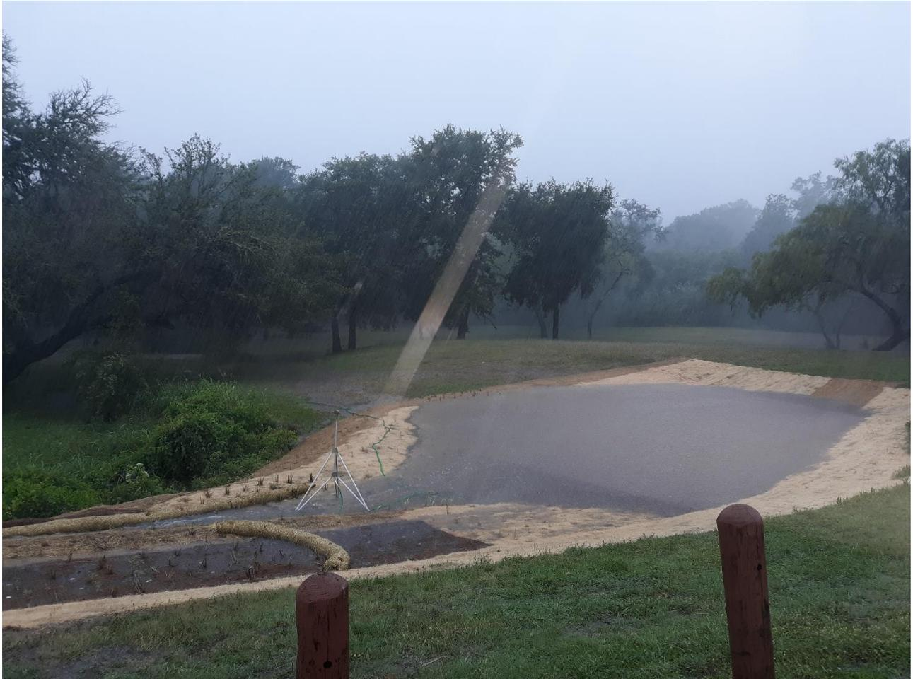
*Fig 9. A few days after installation a 4 inch rain fell and City staff captured this image showing approx. 1/3<sup>rd</sup> of the flow from the conduit being diverted into the garden. Slow overtopping occurred, as expected, along the downslope edge of the bowl. Once the planted vegetation has developed this area is expected to become more and more stable further slowing over-topping while trapping floating debris.*
